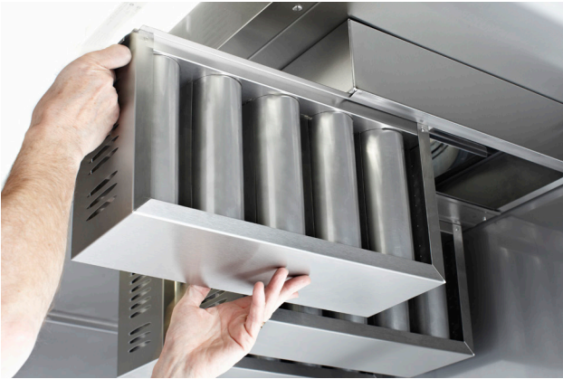
The filter cassette is slid into the filter housing.
